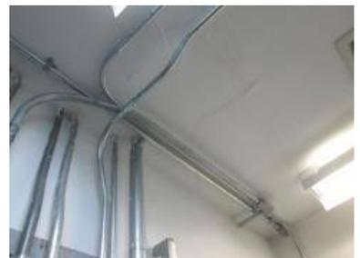
Photo #6: Abandoned wiring in sump.
