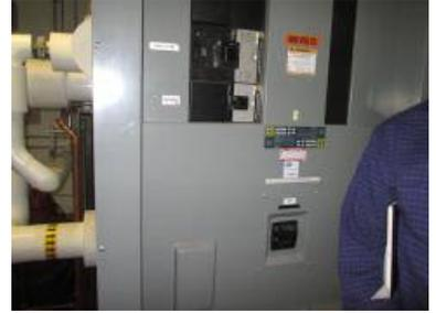
*Photo #2:* Example of interior electrical subpanel with cover off for inspection.
