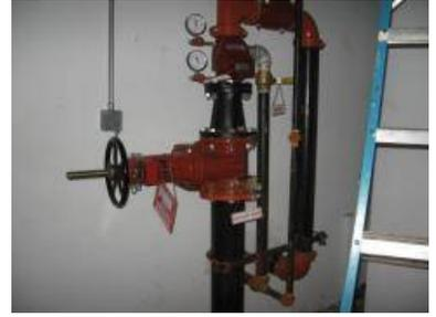
Photo #2: Leak at one valve of sprinkler main valving.
