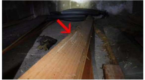
Photo #5: Apparent visible mold: wood scraps in crawl space.
